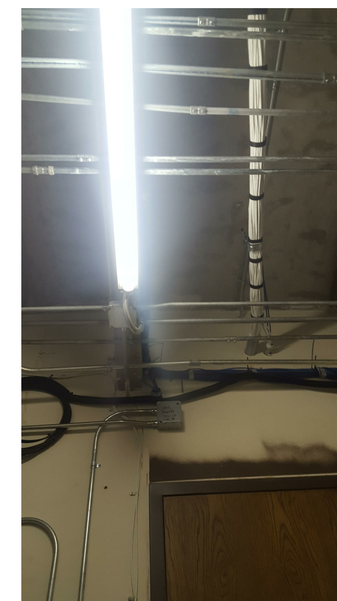
3 EXISTING IDF - SOUTH WALL 1/2" = 1'-0"
