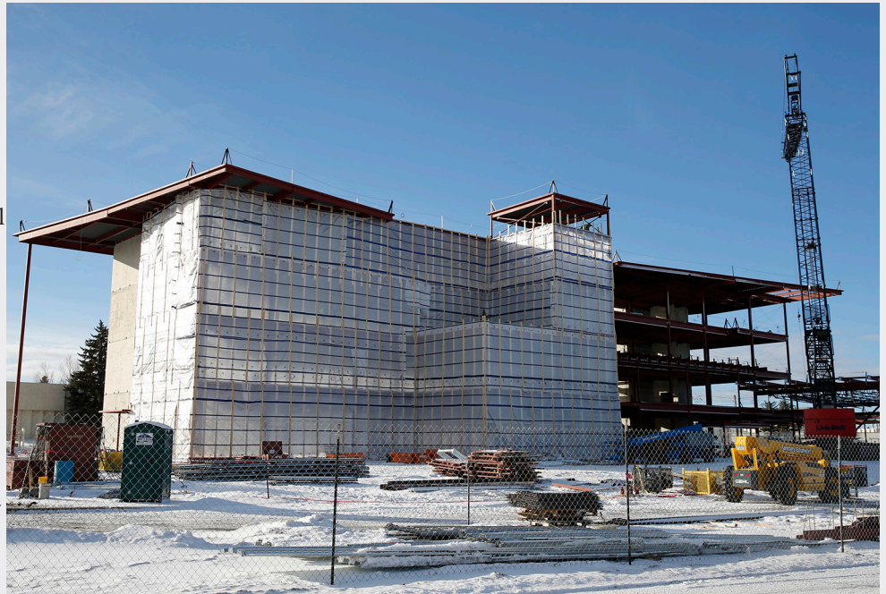
Plastic sheeting encloses the Student Services/University Center as crews work on interior structures. Michael Smith/LCCC
