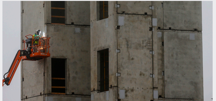
Crews continue work on the Student Services/University Center building. Michael Smith/LCCC
