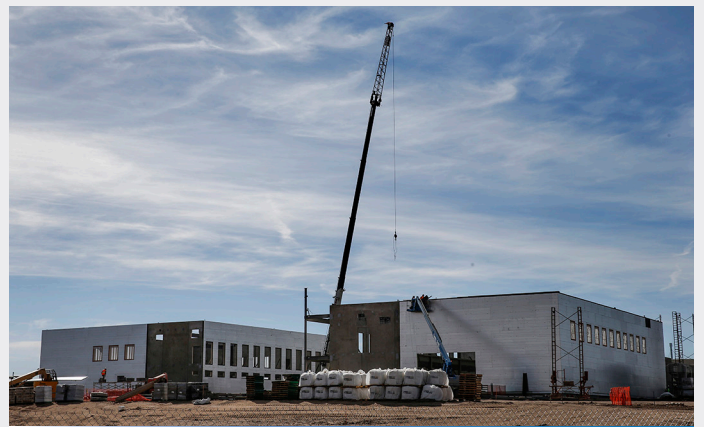
Work progresses on the Flexible Industrial Technology building. Michael Smith/LCCC
